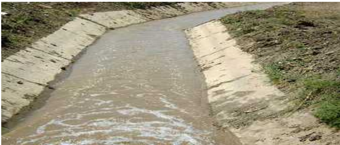
Figure 4 Cemented canals in Lower Kuja irrigation project
